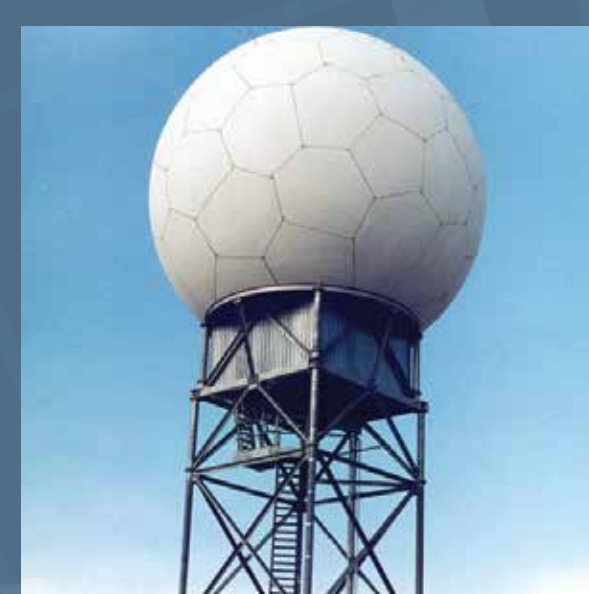
Fixed Weather Radar
